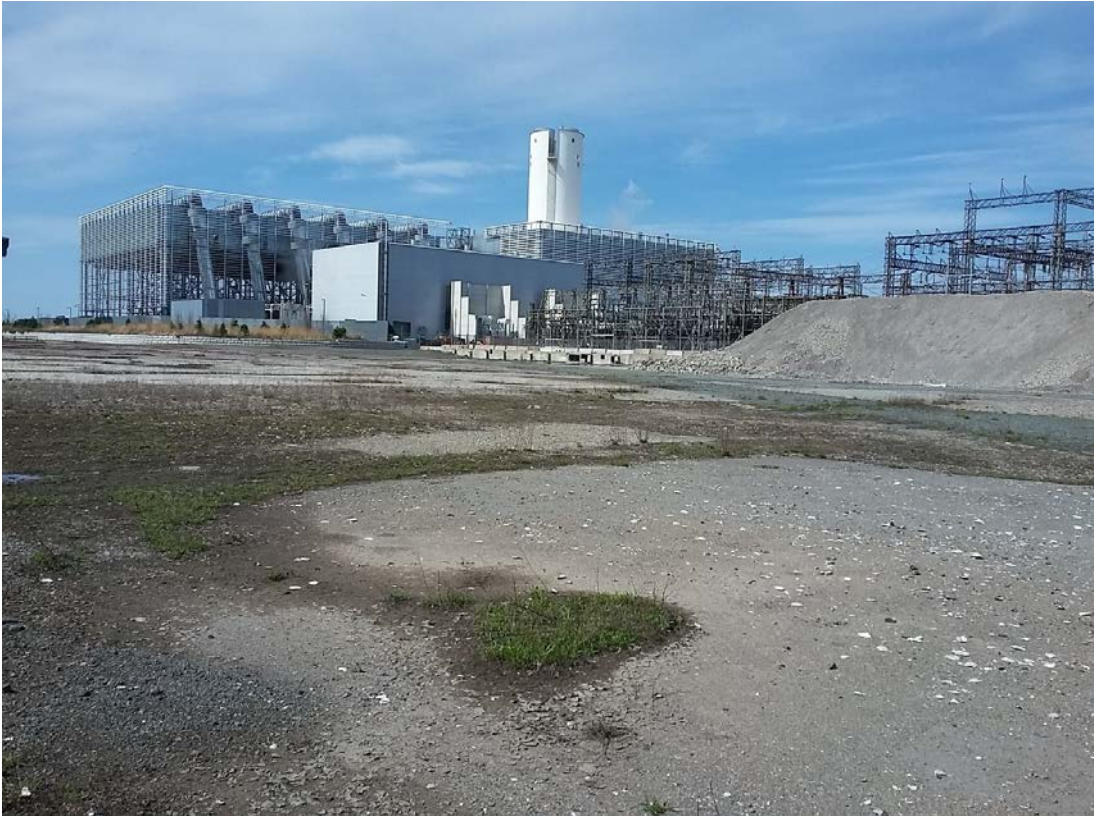
Photo 5: View looking southwest towards the western side of the Salem Harbor Power Development facility
