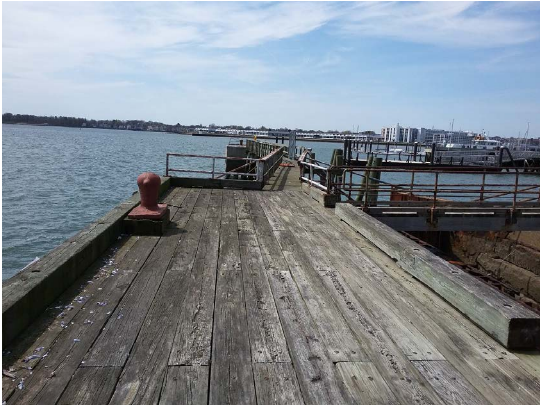
Photo 8: View looking southwest from the southern end of the wharf
