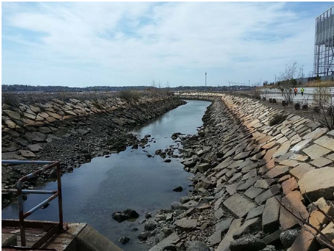
Photo 6: View looking south down the former discharge channel
