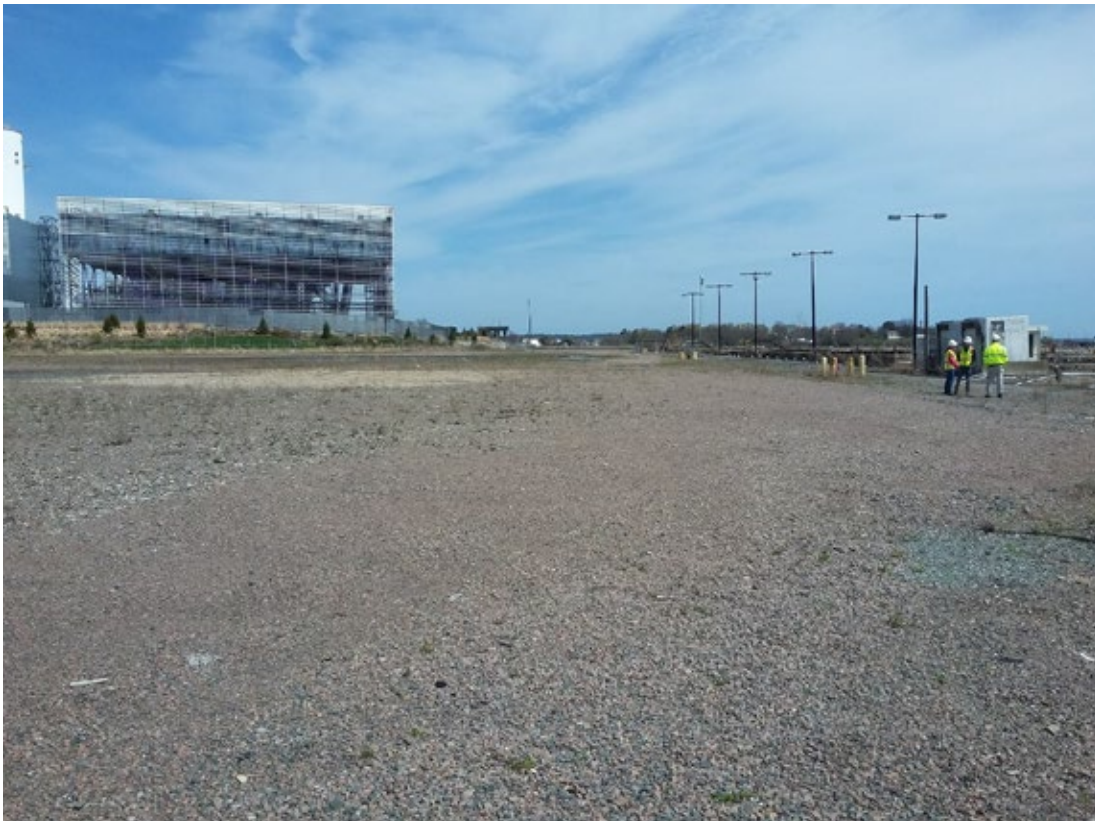
Photo 3: View looking northeast from the southeastern edge of the Salem Harbor Power Development facility
